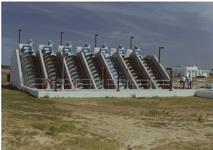
The Archimedean Screw in use at a water treatment plant in Tennessee
